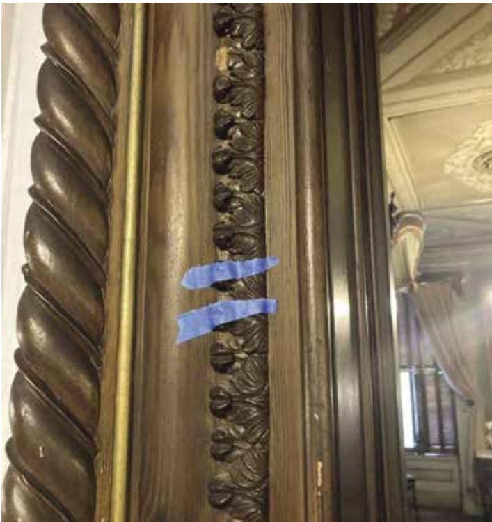
Intern Sylvia Brock's work on re-adhering decoration to Mansion doors.
