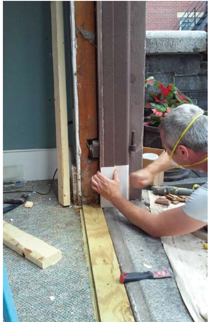
Sebastian Cariddi fitting patch on Carriage House door.
